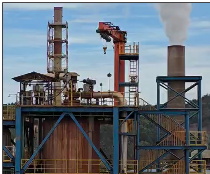
High-pressure acid leach (HPAL) nickel-cobalt mining site.
