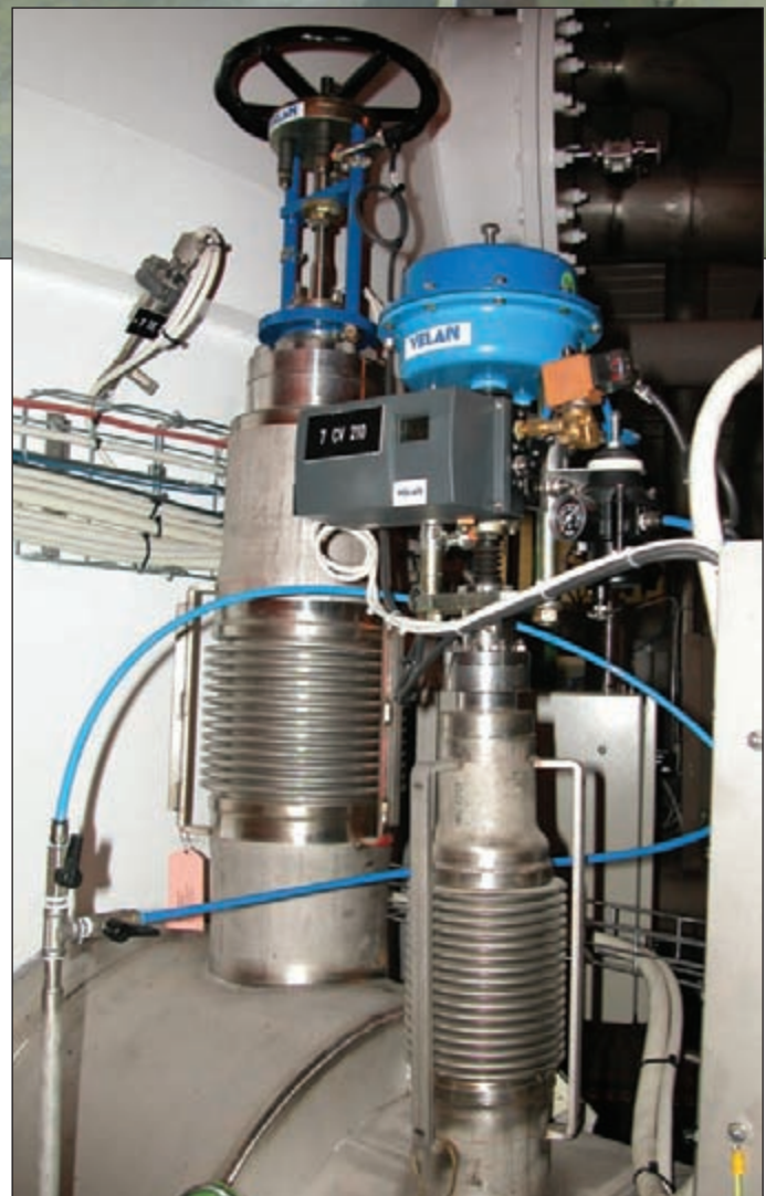
Velan Bellow Seal Control valves with vacuum jacketed insulation installed along the 27 Km accelerator lines.
