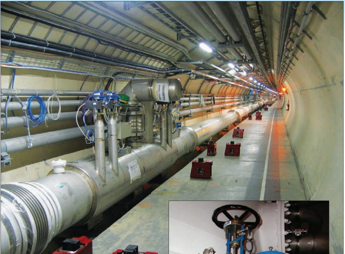
Velan Bellow Seal Control valves with vacuum jacketed insulation installed along the 27 Km accelerator lines.
