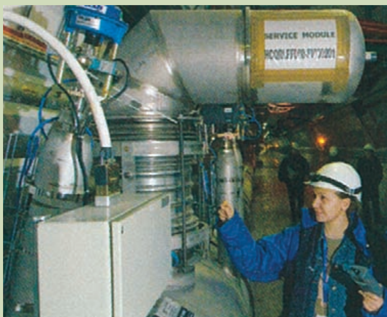
The first section of the cryogenic distribution line, corresponding to an eighth of the accelerator, has been tested at a temperature of 10 K since the end of November 2005.
