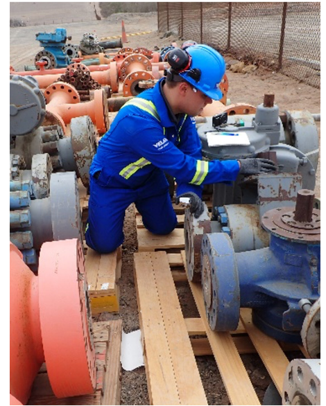
On-site service for Velan valves.
