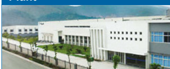
Suzhou, China Velan Valve (Suzhou) Co. Ltd.
